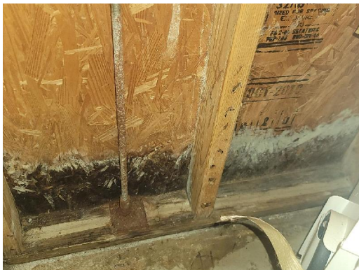
Interior Kitchen South lower wood framing, wall cavity Visible water damage Visible microbial growth
