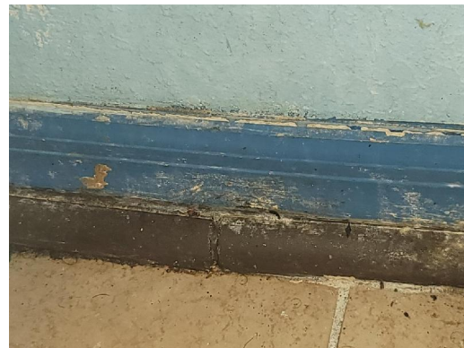
Interior East Bathroom West lower drywall, wood baseboard Visible water damage Visible microbial growth
