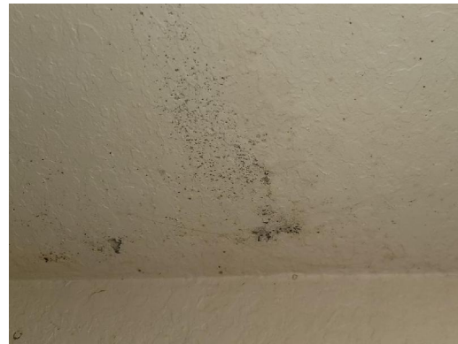
Interior West Bathroom West upper drywall wall, ceiling Visible microbial growth
