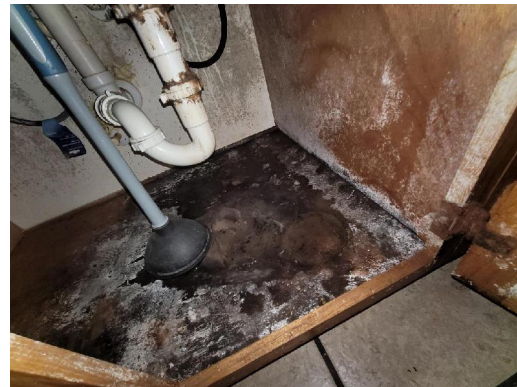
Interior Kitchen Lower wood sink cabinetry Visible water damage Visible microbial growth
