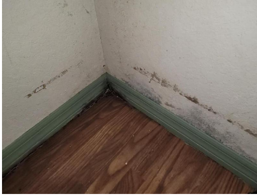
Interior Southwest Bedroom Northwest lower drywall, wood baseboard Visible water damage, standing water Visible microbial growth
